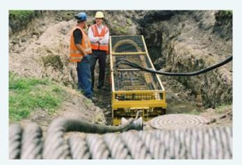
Project Engineer Richard Weaver (right) and a contractor prepare to pull a polyethylene pipe through Hunua No. 1 Watermain using a custom-made winch.
