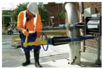
Plant Operator Nigel Prentice opens an isolation valve at the Mangere Wastewater Treatment Plant using a valve-exercising ratchet designed by him and Shift Engineers John Sutherland and Allan Julian. Their tool makes the opening and closing of these valves easy, whereas it used to take time and muscle power. The innovation was recognised with a Continuous Improvement Award.
